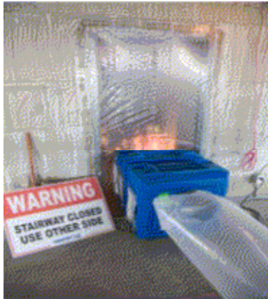
Poly enclosure with HEPA “negative air” unit
